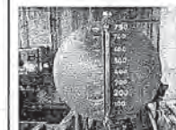
Item No. 2.5 Check diesel level of Engine
