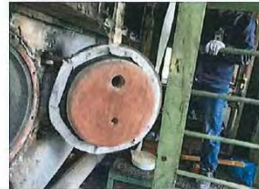
Reversing chamber - smoke tube 2 nd pass
