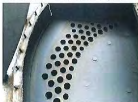
Rear end plate - smoke tube 3 rd pass
