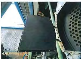
Rear door - smoke tube 3 rd pass
