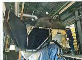
Front reversing chamber – Front door
